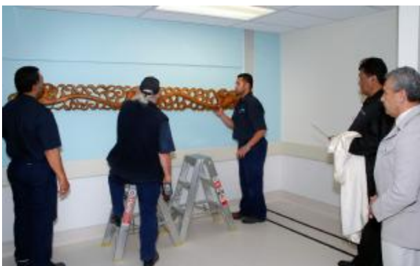
The carpenters re-install the carving
