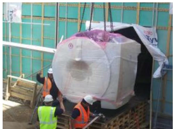
The MRI magnet is lifted into the new MRI Suite
