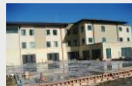
The floor slab is in place
