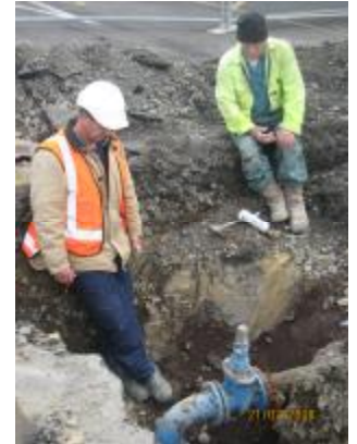
Assessing underground services
