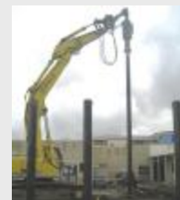
Screws piles are being installed for Buildings A, B & C.
