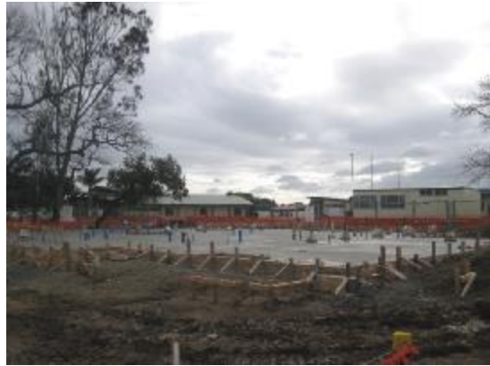
The concrete has been poured for the floor
