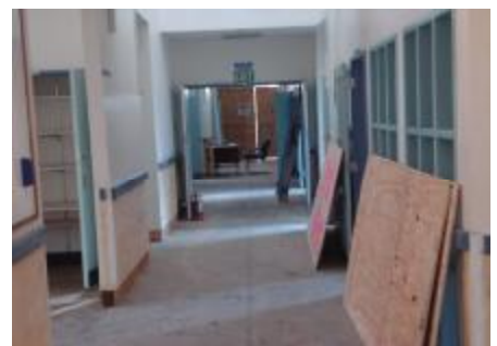
Demolition works are complete. This photo shows the old female wing.
