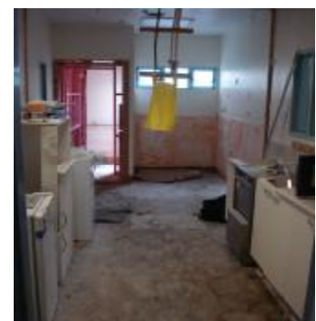
The kitchen has been expanded.
