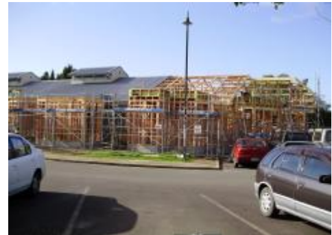
Extension of the General Ward Block
