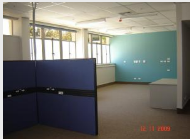
One of the new Radiology Offices
