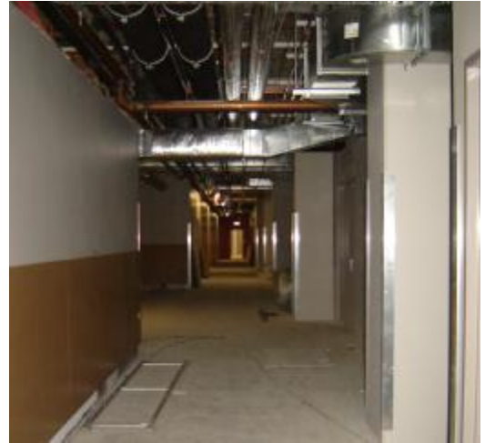
Basement: East wing corridor
