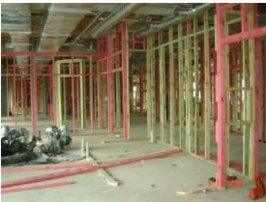
Level 2: Framing of bedrooms
